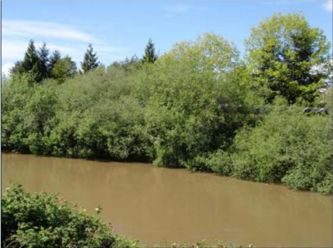
Christiansen Road Levee Bioengineered Levee Repair, Spring 2010.
