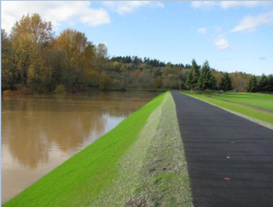
Kent Shops-Narita Levee, Green River, Kent, WA 2010
